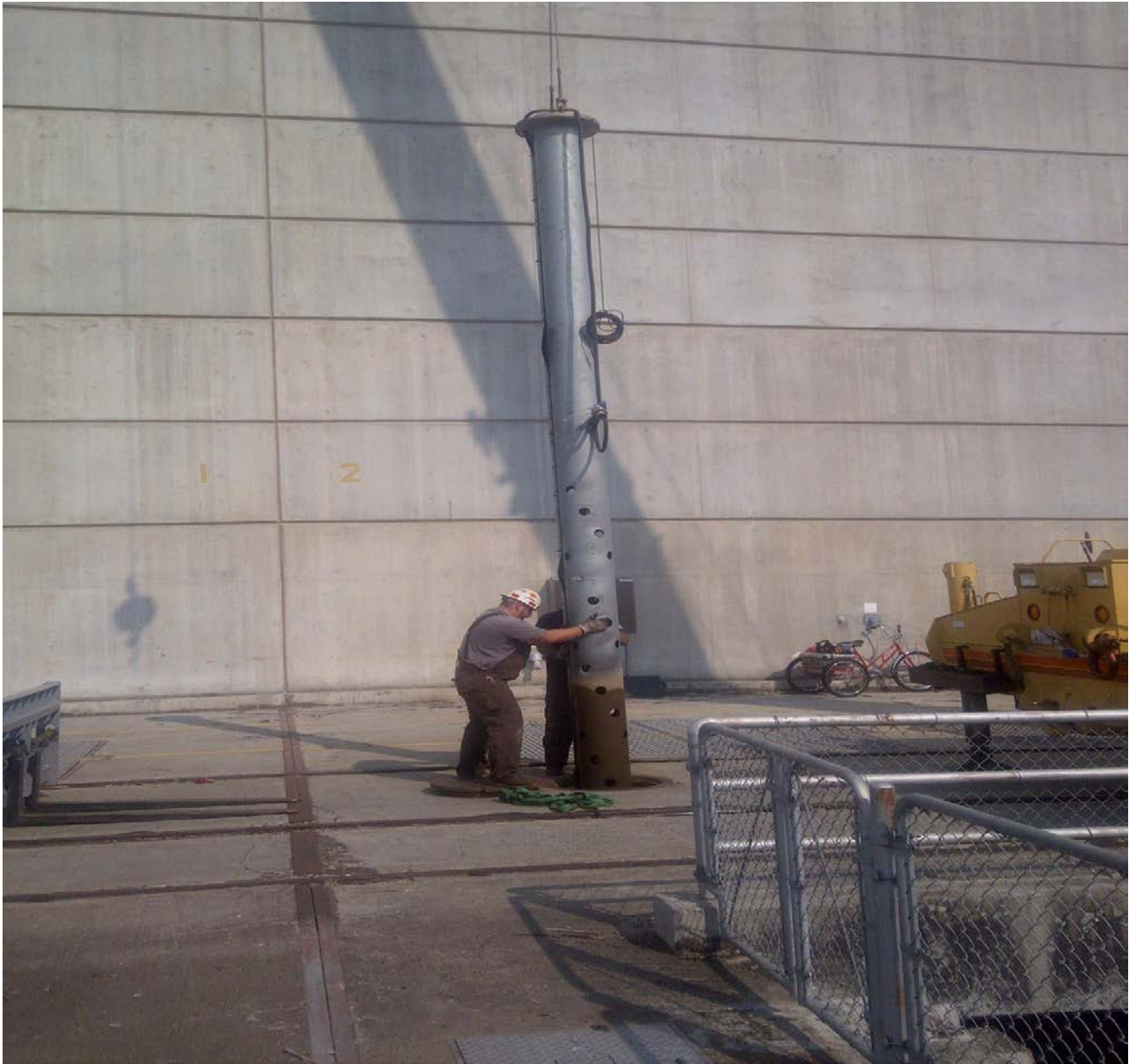
Removal of failed collection channel dewatering pump. One of 10 total pumps.
